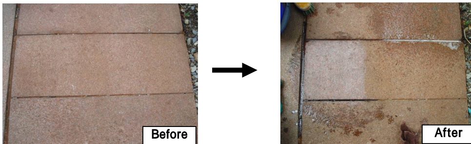
Rust dirt to which iron filings of granite adheres
